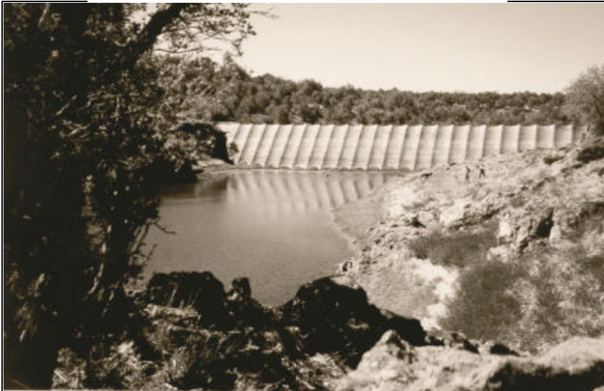
Ashfork Bainbridge Steel Dam
